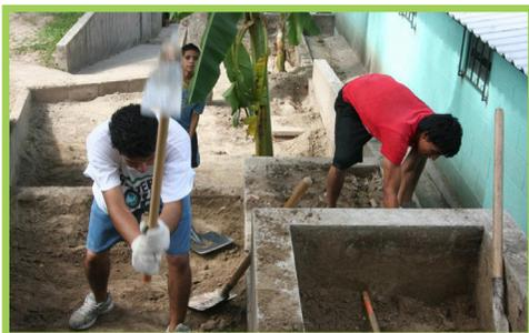
harvesting systems. Each system will hold 14,000 gallons of water, which will be collected through guttering and downspouts on the buildings' metal roofs. The project is underway, with men digging by hand the two large holes to contain the water – one at each of the buildings. Both systems should be complete and operational in time
